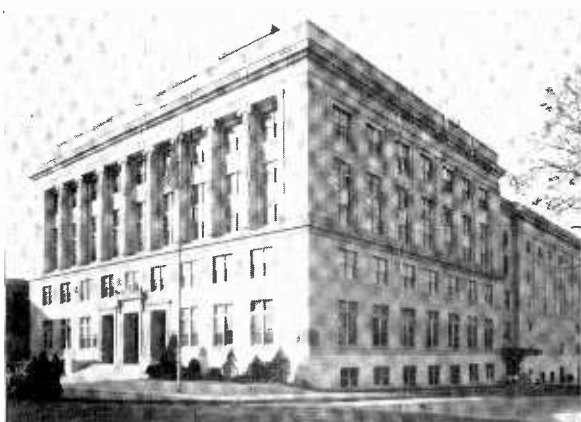
1923 As soon as it became possible to "pipe" programs from locations removed from the transmitter, WKY's studio was moved to the roof of the Shrine Temple and the transmitter to Packingtown.
