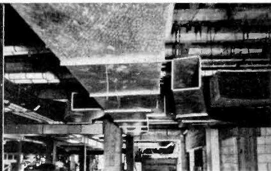
Views of part of the air conditioning equipment and the complicated network of ducts, now hidden above the ceiling, required for the circulation of conditioned air in studios and offices.
