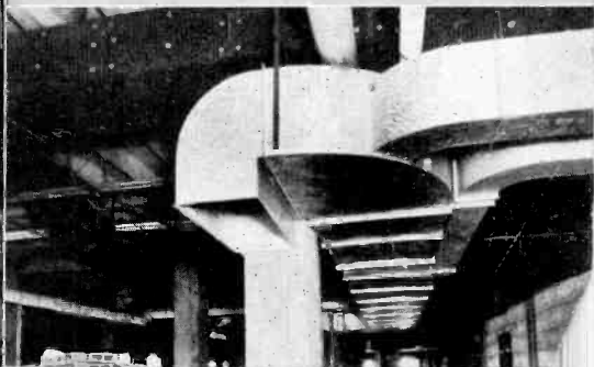
Views of part of the air conditioning equipment and the complicated network of ducts, now hidden above the ceiling, required for the circulation of conditioned air in studios and offices.
