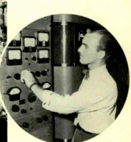
After servicing Sonar equipment in the Navy Harry Wingerter joined the staff of WKMH. He is shown here adjusting the phasing equipment which controls the station's four tower array.
