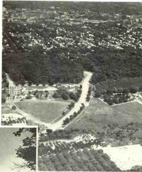
The site of the Veteran's Hospital from the air.
