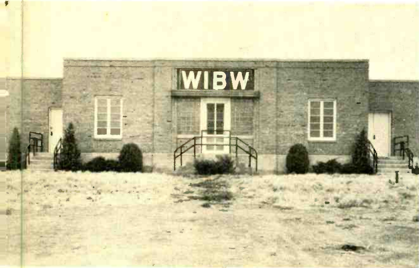
WIBW's new Transmitter Plant building is located in the bottom land of the Kaw Valley. Here, radial ground wires extend over 62½ acres to assure perfect transmission from our lofty 445 foot antenna mast.
