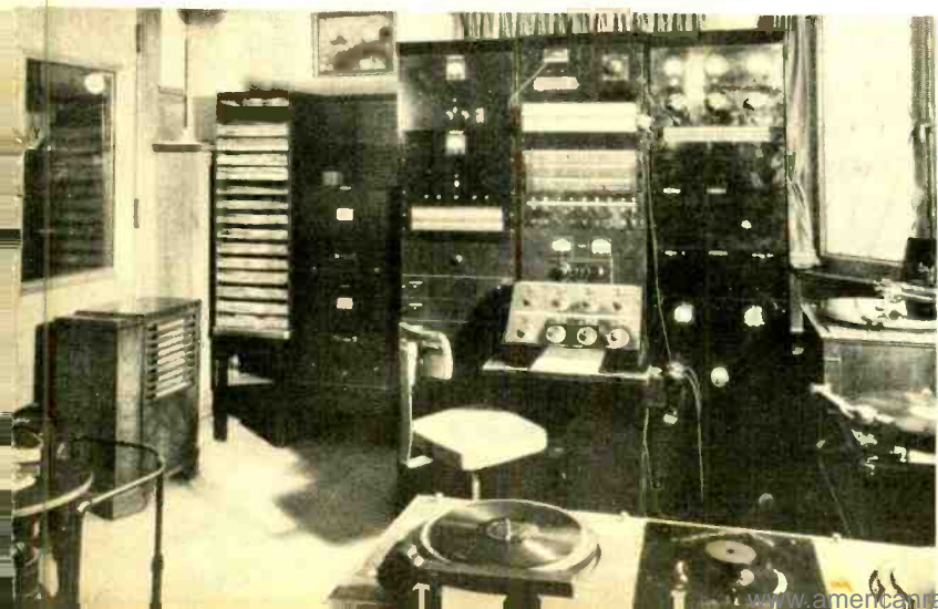
Master Control Room at our Topeka home-studios was once Senator Capper's den. From it one has a view of either studio. The "mixing panel" in the center of the tall rack is the point from which all local programs are regulated.
