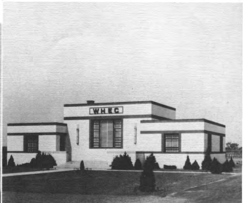
An exterior view of the beautiful WHEC transmitter building on Mt. Read boulevard with the towering antennae reaching skyward.
