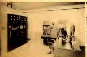
NEW TRANSMITTER was erected near Cook Paint factory in North Kansas City, in 1930. A 1,000-watt Western Electric set; licensed to operate daytime only with 500 watts.
