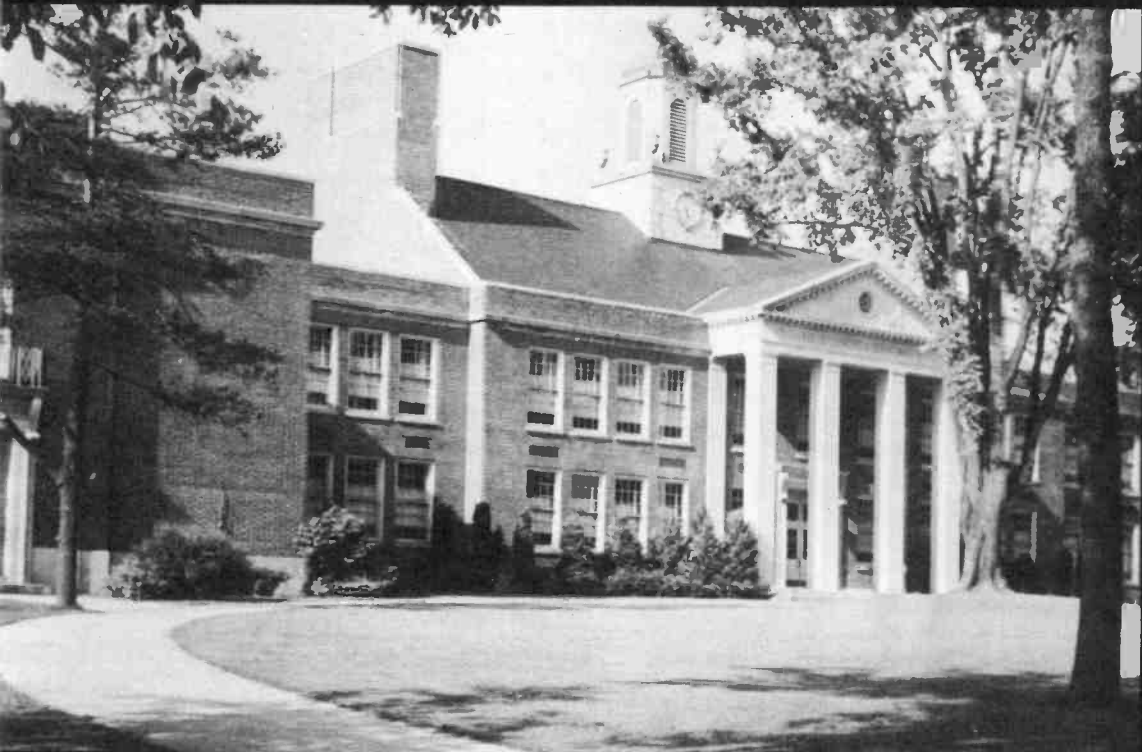
WGY recommends the use of the best educational facilities for farm youth
