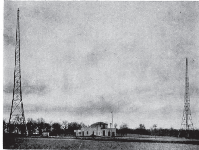
The hopping-off place. Programs are carried by wire from the studio in Chicago to the transmitter in the Spanish bungalow near Elgin. The steel towers, which support the antenna rigging, are 250 feet high.
