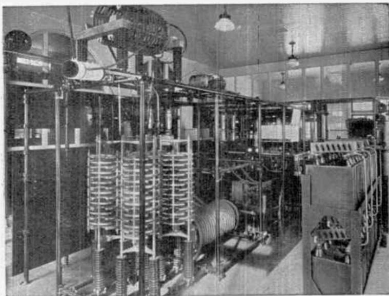
*Spick and span as mother's kitchen range! A rear view of the W-G-N transmitting equipment at Elgin. In the foreground are the helix, condensers, and the end of a block of batteries. Isn't that a dandy helix!*
