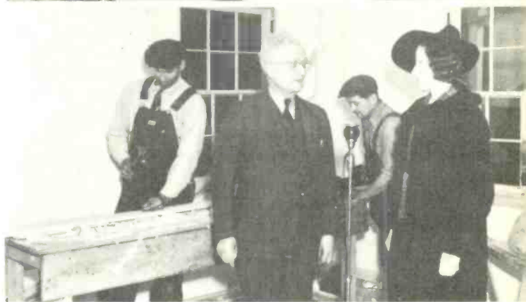
Above—Throughout construction of "Radio's Model Home" being built in downtown Cleveland by the Cleveland Low Cost Housing Association, each step has been relayed to WGAR listeners. In the photo are: Miss Murielle Reid of the Builders' Exchange and Mr. R. L. Hawkins of the Cleveland Paint, Varnish and Lacquer Association during a broadcast interview.
