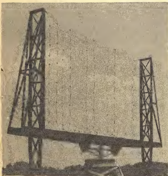
The antenna of the first complete radar, installed 'topside' a building at Naval Research Laboratory in Anacostia, D. C. It is mounted so that it can be turned to allow for around-the-compass search.
