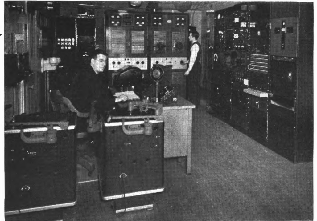
The Control Room with Engineer Seibold on duty.
