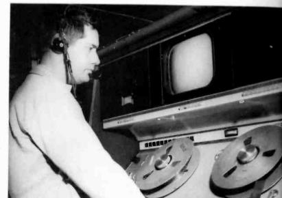
WFBM has always acquired the latest in electronic assistance for a more efficient operation. Engineer Arthur Smith operates the most recent acquisition, a video tape machine in the new television remote unit.
