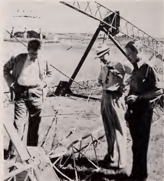
High winds reaching 80 miles an hour levelled the smaller of two radiators at the KFVR (Bismarck, N. D.) transmitter.
