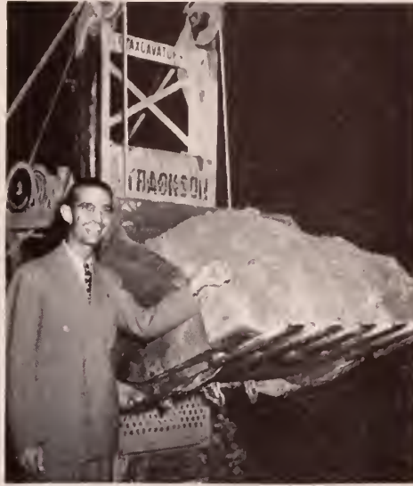
FIRST SCOOP—There's plenty of reason for the big grin on the face of Karl Wylar, manager of Station KTSM (El Paso, Tex.). He's fondling a part of the first shovelful of dirt from the site for the new KTSM building, now under construction. Ground-breaking ceremonies for the new structure were held on the station's 17th anniversary. The new building, of modified Spanish architecture, will be located in downtown El Paso, at the corner of North Oregon Street and West Yandell Boulevard. The broadcasting building is expected to be ready for occupancy in the Spring of 1947.
