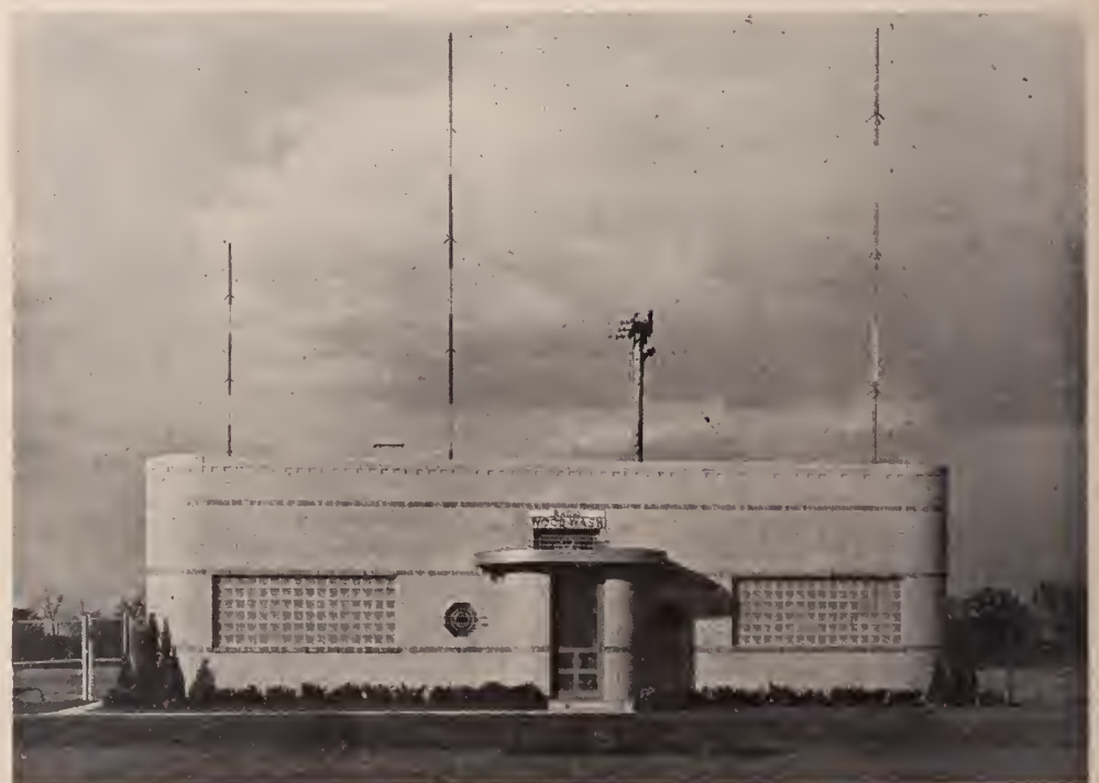
MODERN AND POWERFUL—Here's the new building housing WOOD's 5-kilowatt transmitter. The structure has many engineering innovations.
