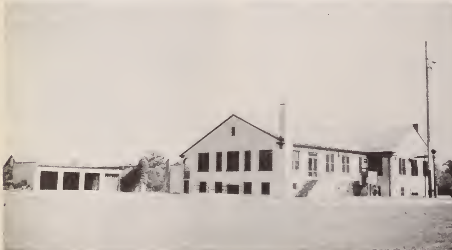
The home-like structure that houses the transmitting equipment of Station WEAF in Bellmore, Long Island. The picture was taken by Robert Covell of the N. Y. Music Research Division during a recent visit to the station.
