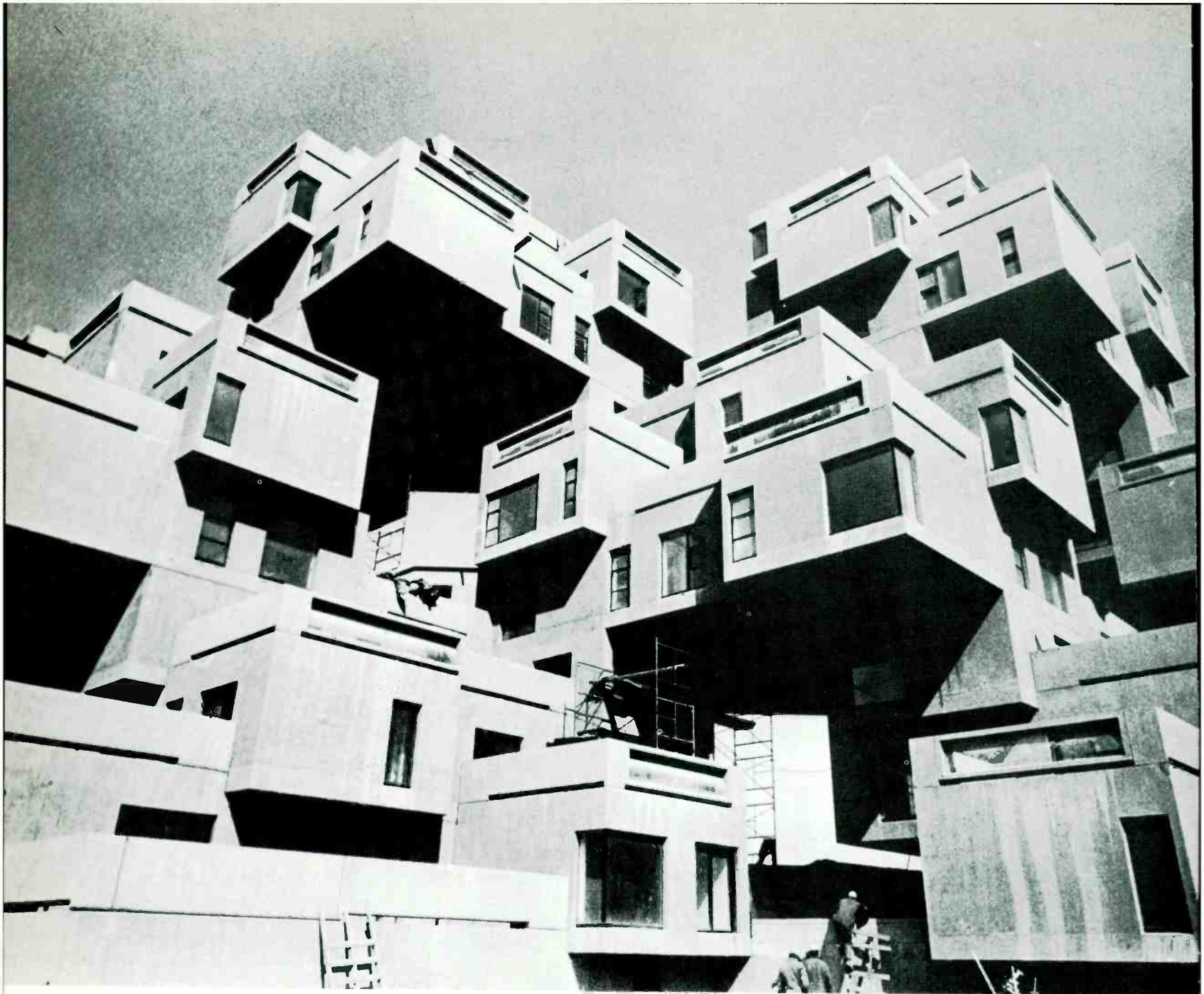
One answer to the population explosion—and it resembles early cliff-dwellings. At Expo 67 it was called Habitat. Its basic unit, a precast concrete block that is finished off with windows and utilities. Architect Moshe Safdie uses the roof of one unit as the patio of another.
