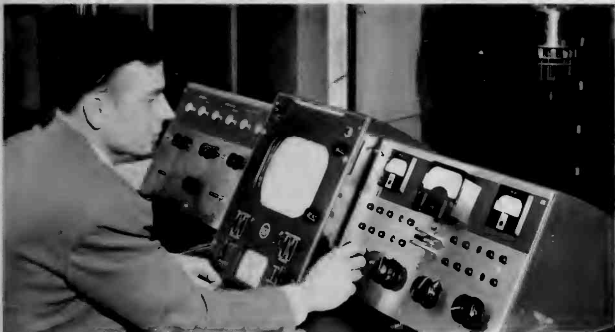
Victor Bary at control console and transmitter switchboard.
