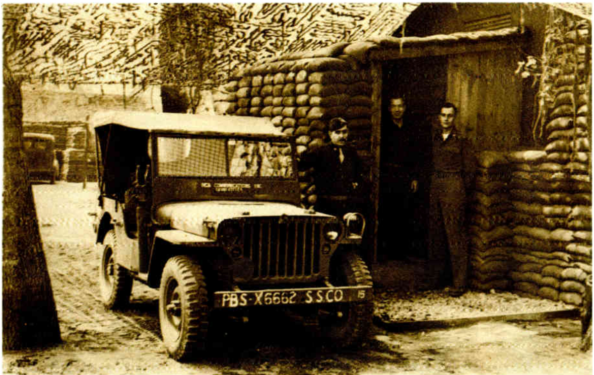
Operators of R.C.A.C. at the sandbag-protected front door of the radio station they established at Naples — the first all-American-owned and operated commercial station in Europe, which went on the air February 1, 1944; a second RCA station opened on June 13, 1944, at Rome.
