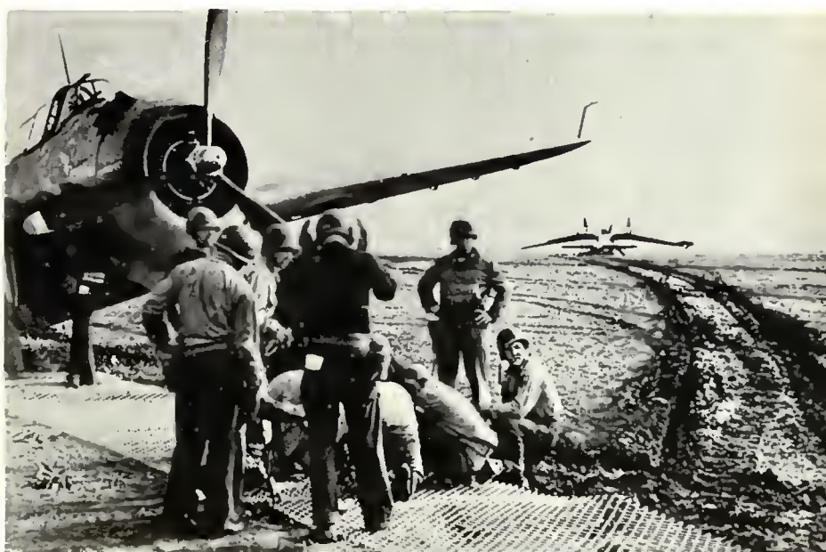
Seabees build landing fields on muddy wastes
