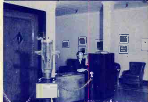
4th floor lobby - Maebelle Pearson at switchboard and reception desk.
