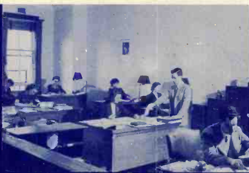
General Office -- 4th Floor rear.
