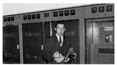
At left, chief engineer Don Burrichter in front of the KMA transmitter at the KMA towers, looks over two transmitter tubes. Generating extreme heat, the old, longnecked tube is water-cooled, the new model cooled by forced air.
