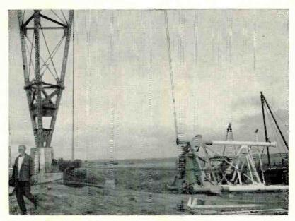
Going Up! The new 670 foot KFYR-tv transmitter tower under construction. In these and the accompanying pictures, one section is shown being lifted into place some 500 feet up...
