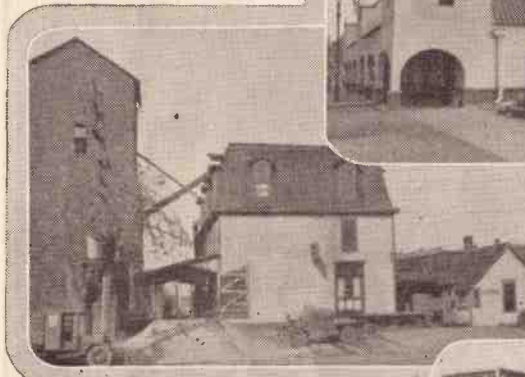
The mill property which we recently got and will probably remodel as soon as possible to make it fit our needs.
