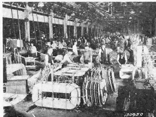
Winding huge coils, Main Works of Westinghouse Electric & Manufacturing Co.
