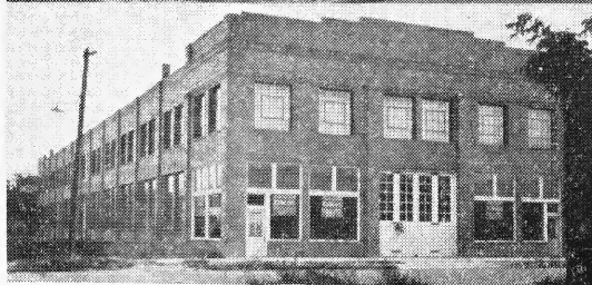
ABOVE—The Stitt Building, with Chamber of Commerce and KFKX Studios on Second Floor. CENTER—Swift & Company Produce Plant, just completed. BELOW—The Smith Machinery Company Building.
