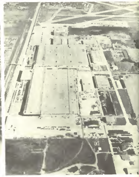
An aerial view of Chance-Vought Aircraft gives an idea of the tremendous task on hand when the company decided in 1948 to move its plants from Bridgeport, Conn., to Texas. More than 1,000 freight cars were required to move the 27 million pounds of machinery. Thirteen hundred employees joined in the trek to Dallas.
