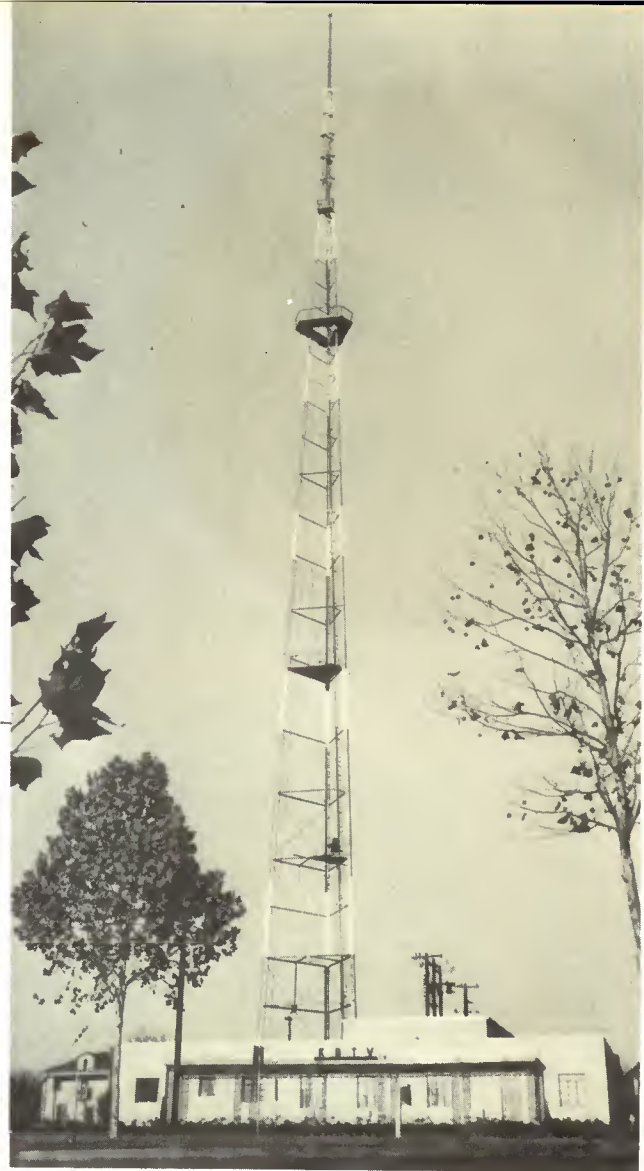
Here is a side view of KBTv with its lofty self-supporting IDECO antenna tower in the background.
