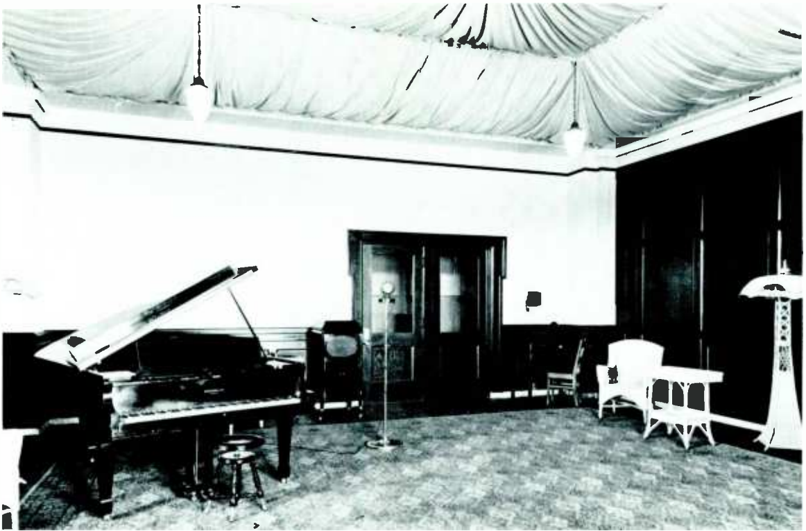
CNRV's studio was housed in the Vancouver CNR depot. The ceiling is hung with sound-absorbing material. (Leonard Frank photo)
