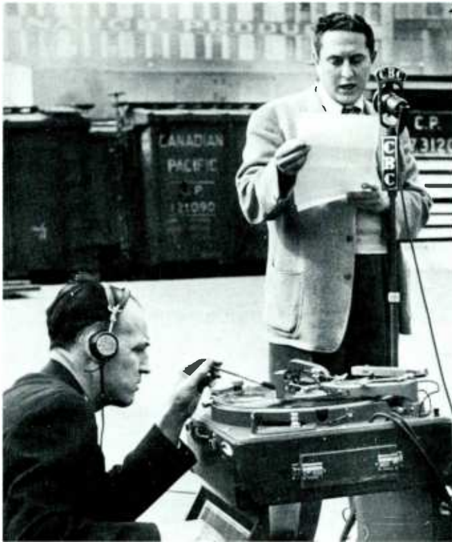
Announcer Bill Herbert recording a program "in the field" with technician Clayton Wilson in the 1940s. Herbert's commentary is being recorded on a Model Y disk recorder; Wilson is ensuring that the strands of cut acetate do not foul the cutting stylus.
