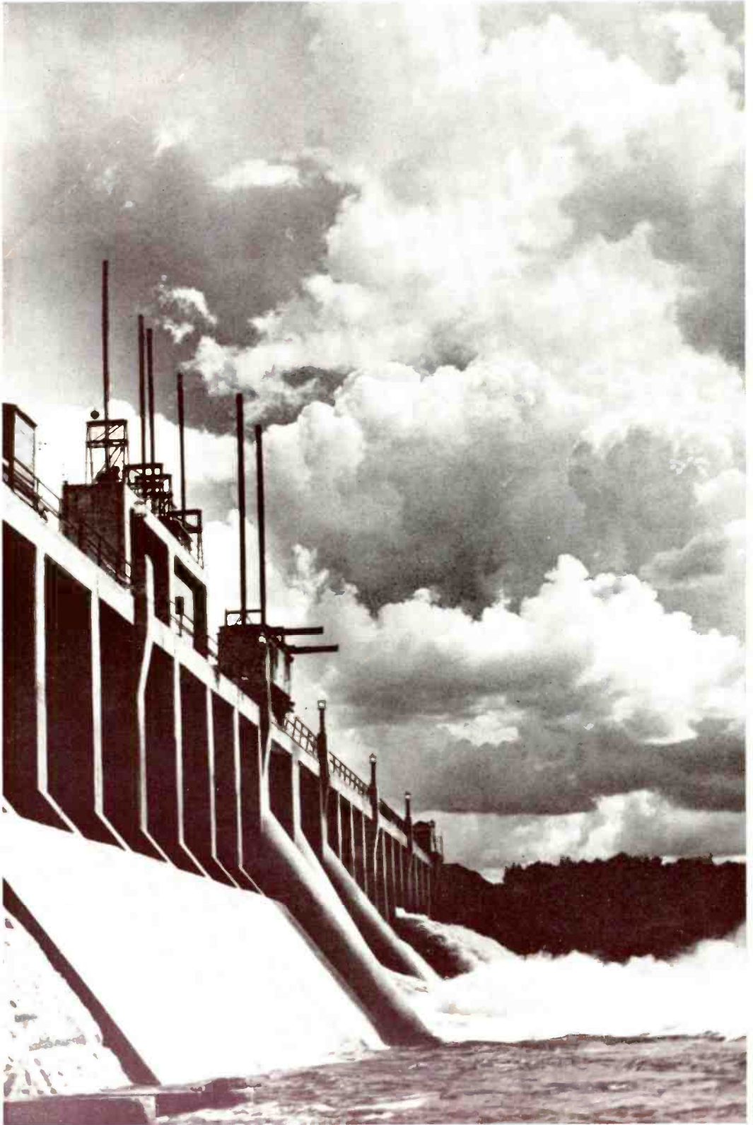
Power Dam at Seven Sisters Falls
