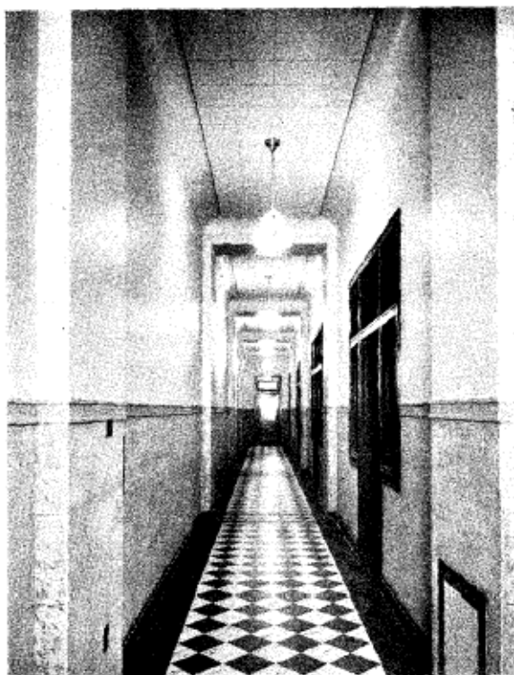
One of the corridors separating CKY Offices from the Studio Block.
