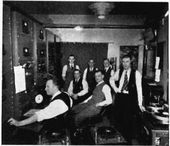
CFRB MAIN CONTROL ROOM
