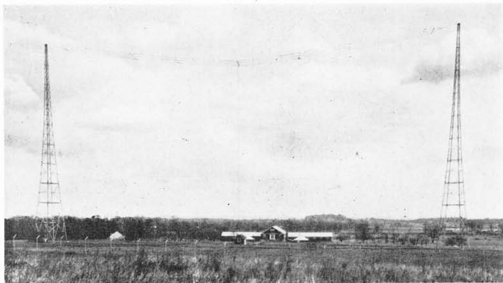
General view of the Whippany Station, 3XN
