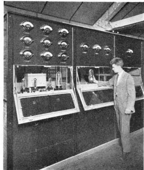
The first three panels of the transmitter
