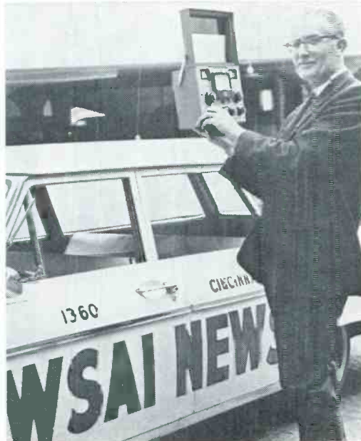
(ABOVE) Engineering progress is vividly illustrated in comparison of mobile units employed by Cincinnati station in late 20's (l) and currently. Chief engineer Vern Milton (r) is holding a compact signal-measuring device which is only a fraction of the bulk of the "field intensity measuring set" of 40 years ago. (WSAI)
