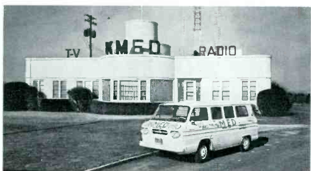
(ABOVE) Compact stations give full radio/tv service to smaller communities; reflect best of management/engineering efficiency. (KMEQ)
