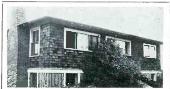
Houses as ordinary as this one on a hilltop near Syracuse, N. Y., served early stations in place of transmitter towers. (WSVR)
