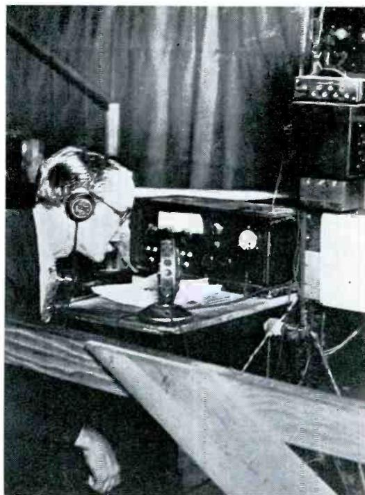
(LEFT) *Before FCC* was created, signals weren't controlled and elaborate, directional antenna was not necessary. Most stations started with a wire strung between two handy points; even a flag-pole would do, as with this 100-watt transmitter which got easy coverage of San Francisco from vantage point above the Bay. (KSAN)
