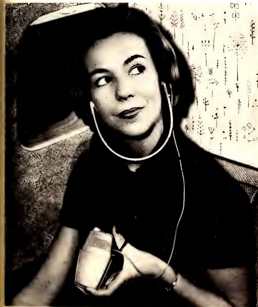
TRANSISTOR radio equipped with earphones provides personal broadcast for each passenger on trans-Atlantic jet flights. Listener pushes button on light-weight receiver to select program
