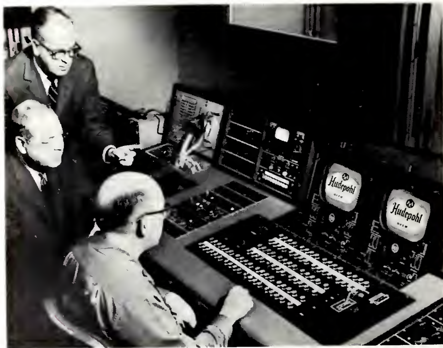
ABOVE, Robert A. McDowell, media v.p. Stockton, West, Burkhart, Inc., watches traffic director type station schedule on Flexowriter. Machine punches out operations tape containing all vital facts for switching cues. BELOW, MacDowell at master control panel. At left is the tape reader into which operations tape is fed. The tape reader interprets the facts, feeds them to a "Univac" type of control which first stores them, then actuates switching of audio and video sources
