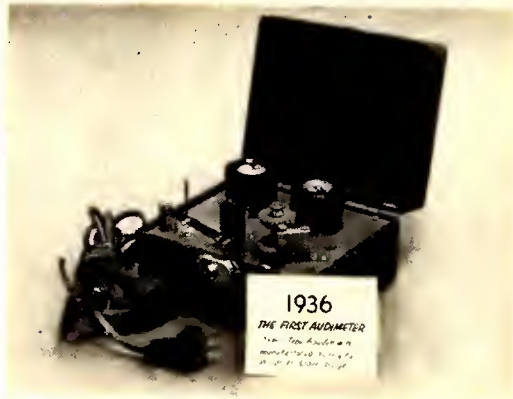
RADIO ERA: Earliest form of checking audience (I) is this "appreciation" post card by Music Master; listeners had to affix their own stamps to vote. In 1936, Nielsen installed its first Audimeters (35 mm tape). Two years later, an improved Audimeter went into radio homes. In 1946, instantaneous radio ratings were shown in Chicago
