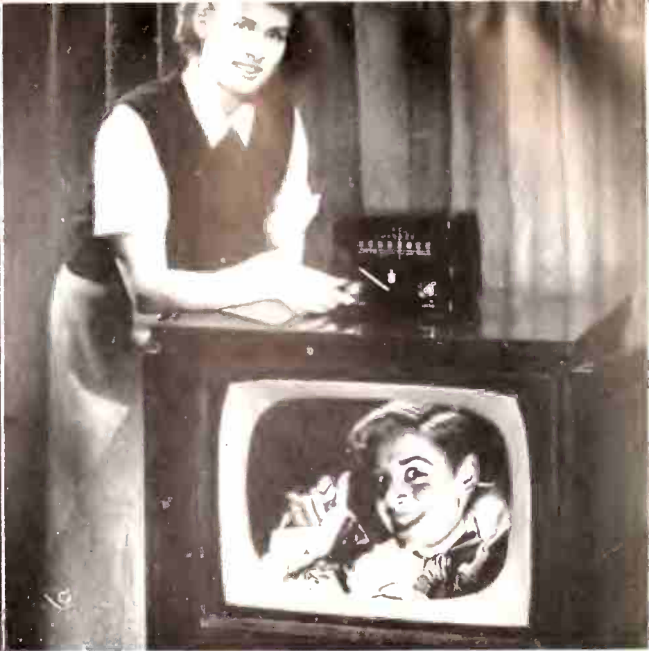
Are converters available? Yes, and production is increasing. Crosley tuner, above, enables VHF set to receive all 83 UHF channels. One- and two-channel converters also are being made
