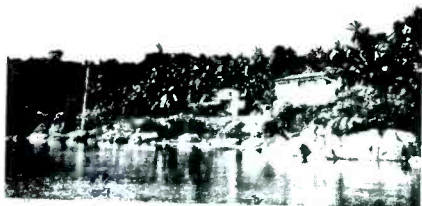
Transmitter Site at Anse Etoile
