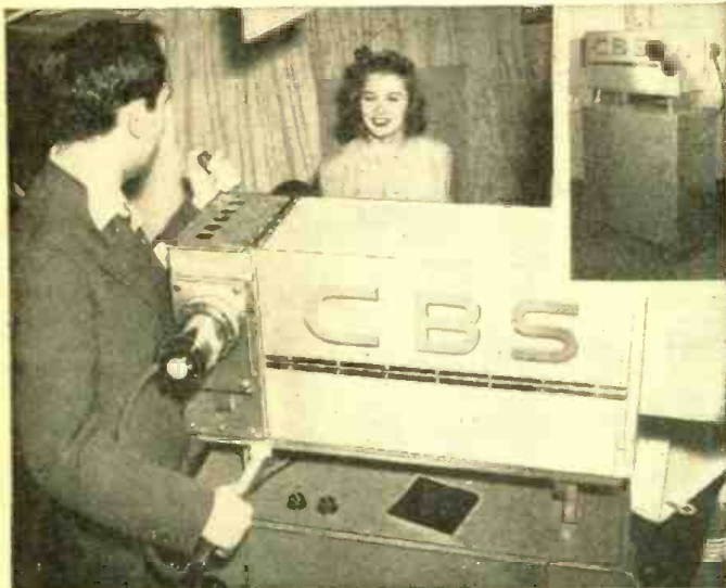
"Engineers'-eye view" of CBS studio during a color television program. This shows rear of apparatus. Insert is front view of equipment, as seen by person being televised.
