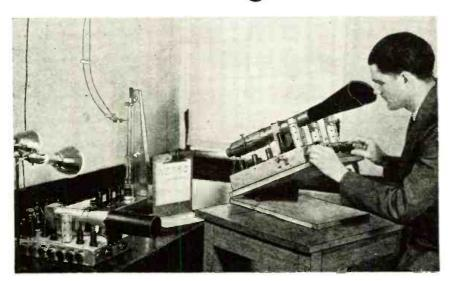
New 2-inch iconoscope opens new field to the radio amateur and the electrical experimenter. Images may be sent by radio or wire.
