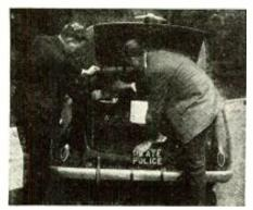
F.M. police equipment installed in luggage compartment of radio car.
