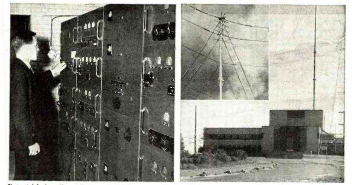
Photo at left shows Harry Whitemore at the transmitter panel of WIXOJ, frequency modulated station at Paxton, Mass. Photos at right show transmitter building at Paxton; 50 kw. equipment under construction. Insert shows transmitter antenna mast, with 4 bay turnstile aerials and vertical aerial on the peak.
