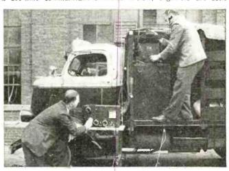
testing the radio equipment on one of the trucks which the expedition includes. A trailer and a cruising sedan will also be employed. The system, powered by standard car batteries, is similar to that used by many police departments. Antennas, ranging from the standard fishpole type to a 128-foot flat-top, are being provided.
