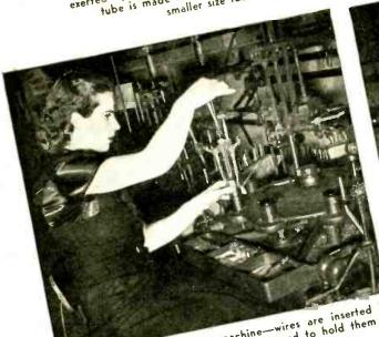
The automatic stem-making machine—wires are inserted in hald them in which is heated and pressed to hold them in The automatic stem-making machine—wires are inserted in in automatic stem-making machine—wires are inserted in the automatic stem-making machine—wires are inserted in the automatic stem-making machine—wires are inserted in automatic stem-making machine—wires are inserted in automatic stem-making machine—wires are inserted in the automatic stem-making machine in the automat
