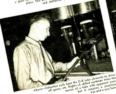
nduction coils heat the C.R tube elements to drive
