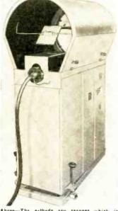
Above—The eathode ray seanner which is installed in front of the speaker. The C. R. tube is mounted vertically and a mirror projects the seanning light onto the subject's face.
