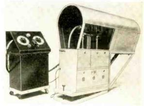
Special television image projector, with control unit at the left. It employs a plate potential of 20,000 volts and a powerful lens projects the image from the left. the end of the tube onto the large screen.
