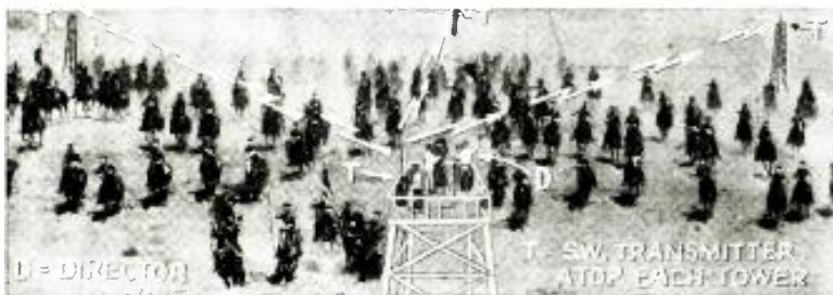
The diagram above shows the great value of short-wave "phone" sets in directing a big movie scene, such as that shown on our front cover and taken from The Charge of the Light Brigade . Not only are the various "camera groups" kept in constant touch with the director-in-chief by short-wave phone, but his aids stationed at various points about the movie lot can be given orders to diminish or increase smoke effects, etc.
