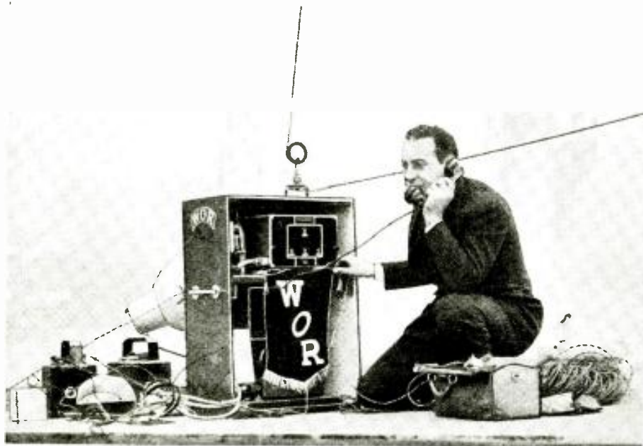
Here we see the operator in charge of the ultra short-wave transmitter and receiver aboard the S. S. Manhattan talking to the land station located in a downtown skyscraper in New York City, from which point the voice was relayed through a wire circuit to the WOR master control room from which point the radio conversations were broadcast over the stations of the Mutual Broadcasting System.
