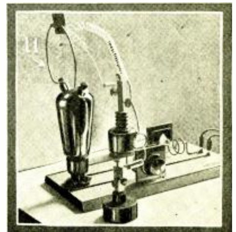
Fig. 5—Transmitter without a support for the block condenser.
