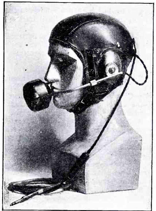
Photo above shows the latest microphone attachment to aircraft pilot's helmet. This device leaves the pilot's hands free and the "mike" can be swung up out of the way when not talking.
