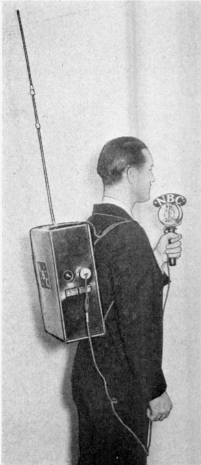
Above—N.B.C. special announcer carrying short-wave transmitter built in "back-pack." Many special events have been relayed on 5 meters from a portable transmitter of this type.
