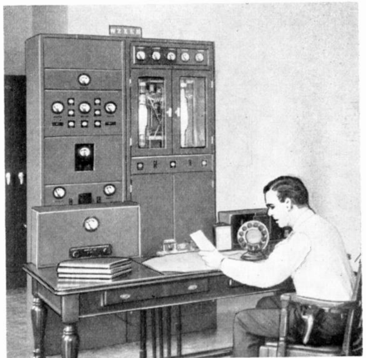
Above—View of the transmission room at Newark Police Headquarters with 50 watt high frequency radio transmitter on left; 500 watt amplifier at right.
