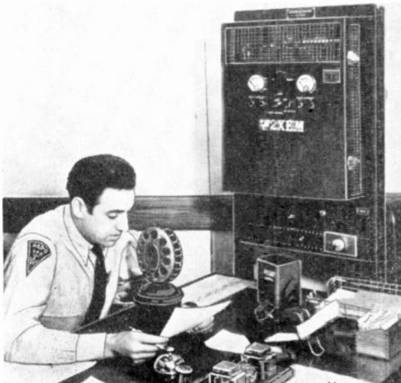
Above—View of the transmission room at Newark Police Headquarters with 50 watt high frequency radio transmitter on left; 500 watt amplifier at right.
