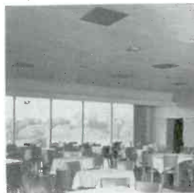
ABOVE: A SOUND-SYSTEM installed by the Hi-Fi Shop. Dark rectangles on the ceiling are built-in bass-reflex speakers.
